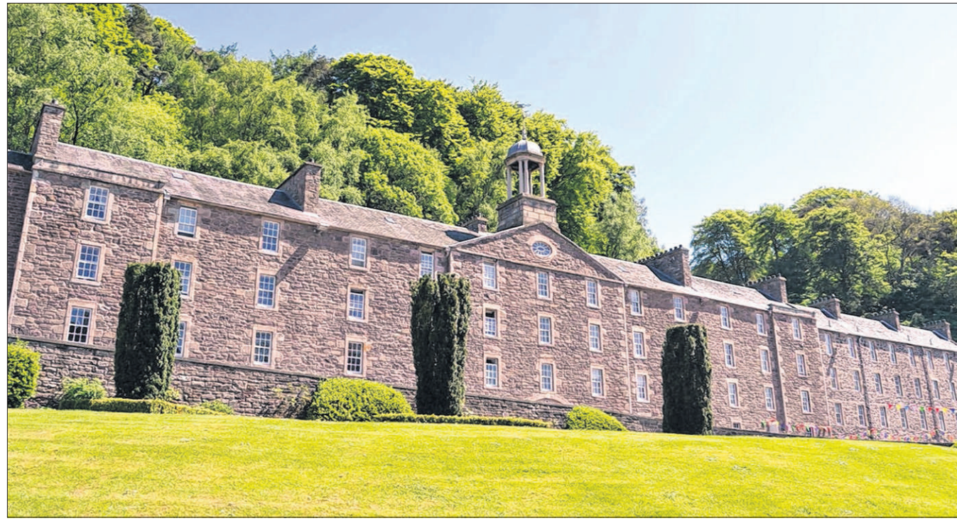
RUN OF THE MILLS: New Trustees are likely to be bewitched by the scale of the UNESCO World Heritage Site at New Lanark.
